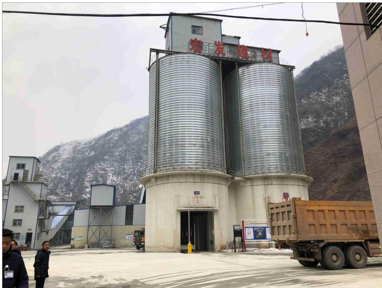
Figure 18.12 Hongfa Aggregate Plant at the Ying site
