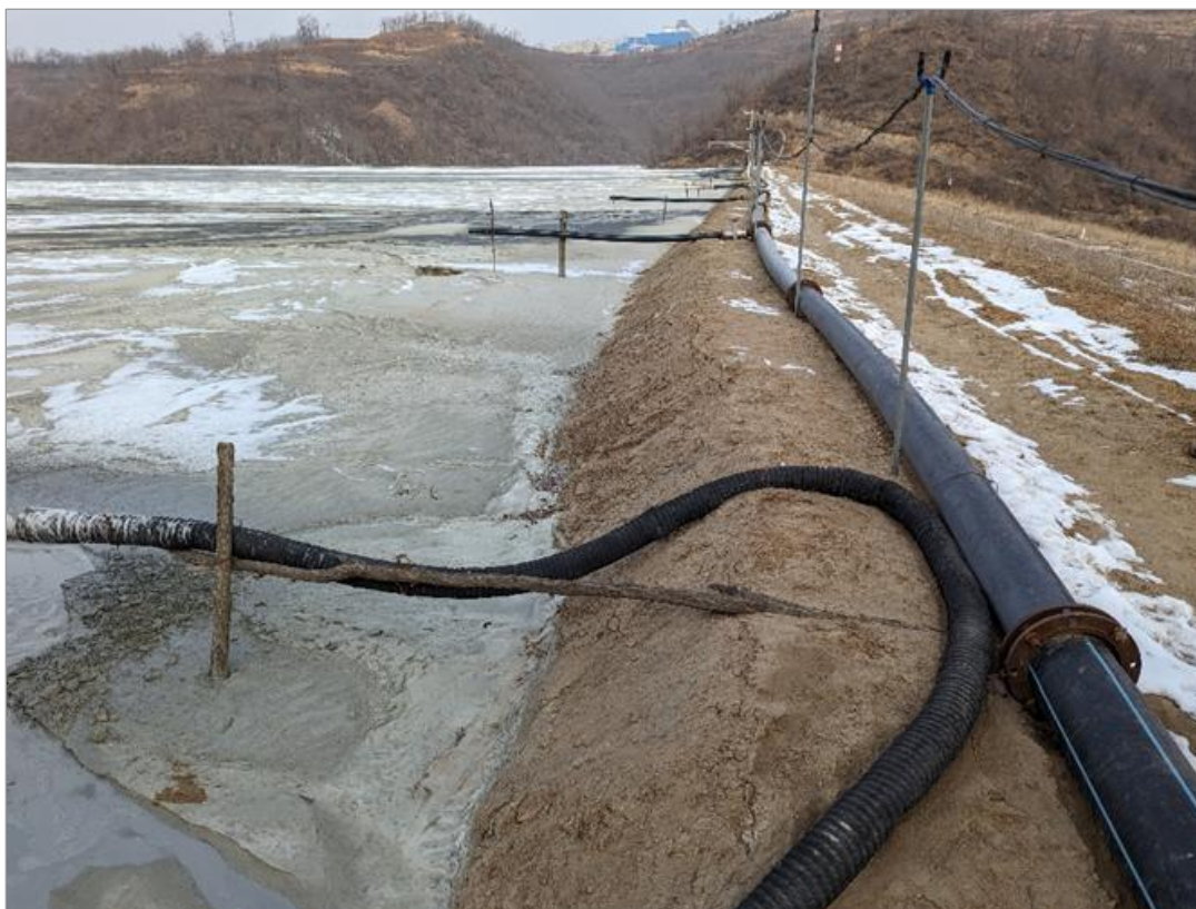
Figure 18.7 Tailings discharge along crest of TSF2
