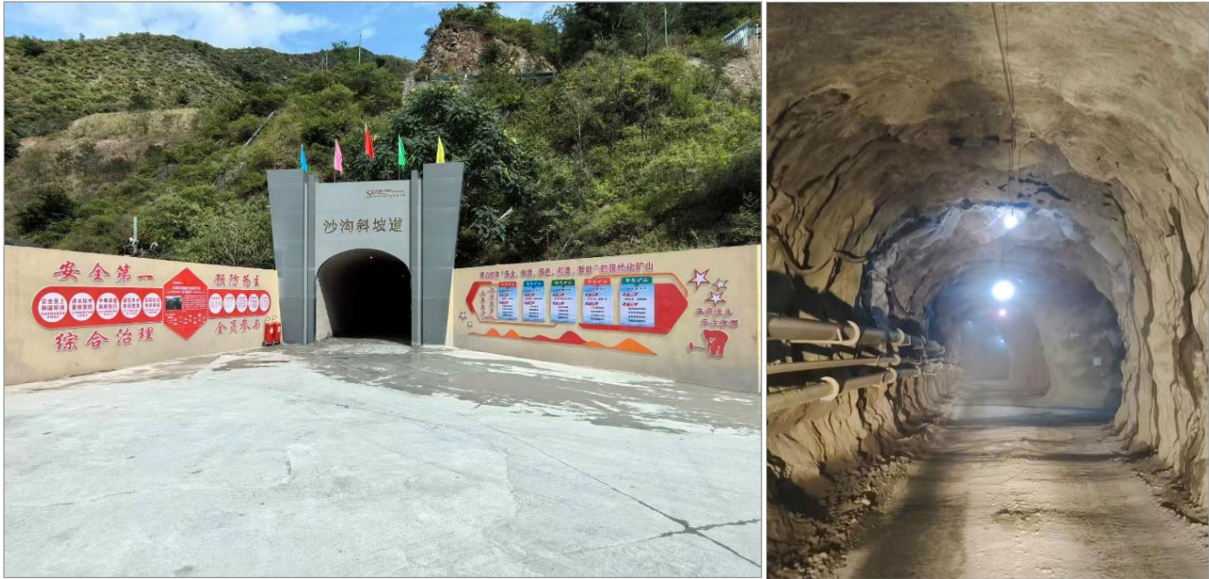
Figure 16.3 Portal and ramp at SGX mine
