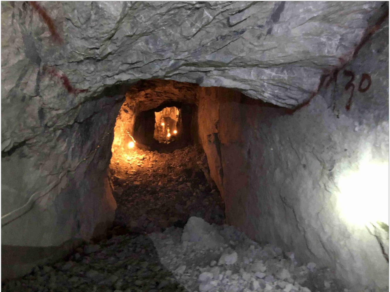
Figure 16.5 TLP mine – A26 shrinkage stope
