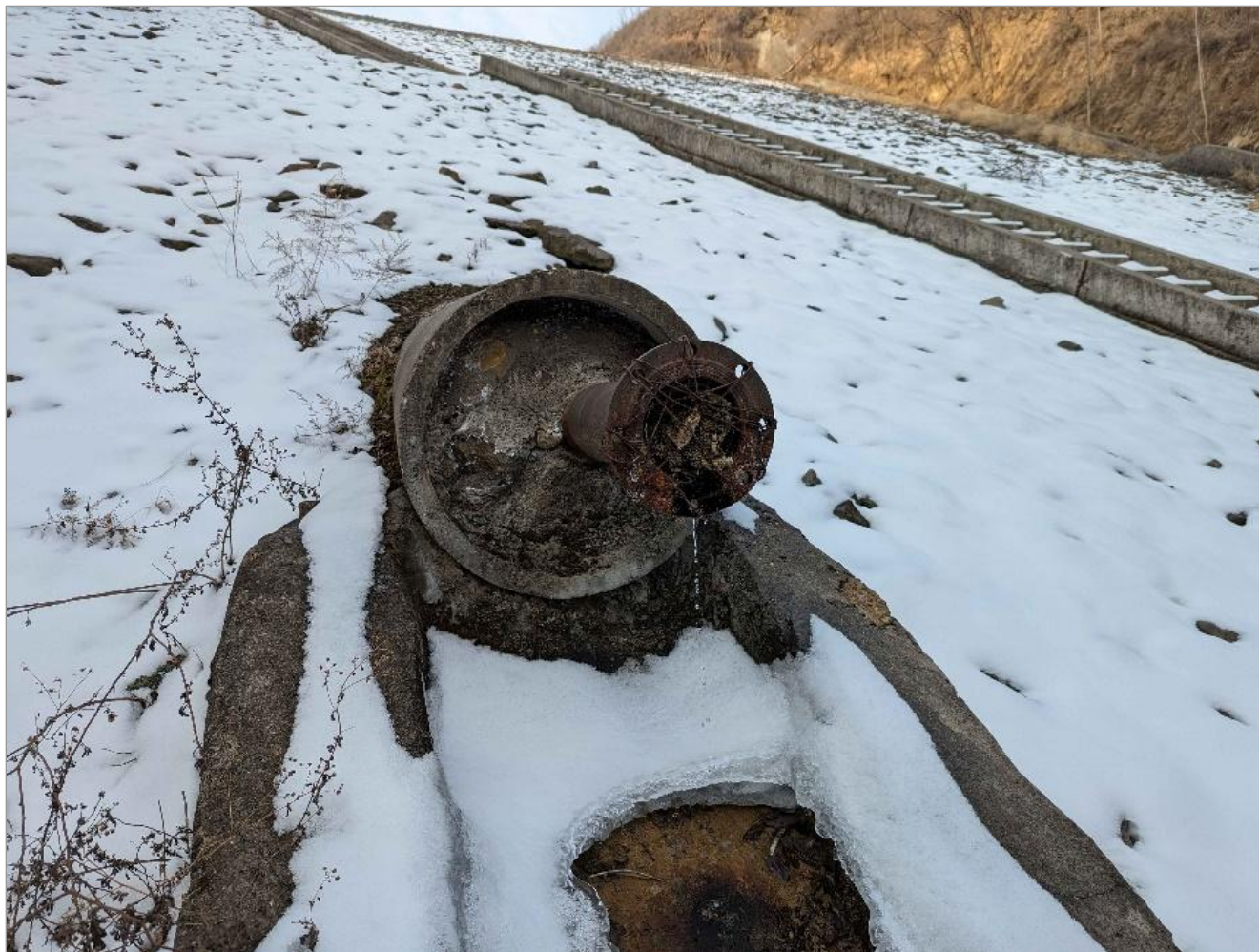
Figure 18.5 Upstream toe drain outlet pipe – TSF1
