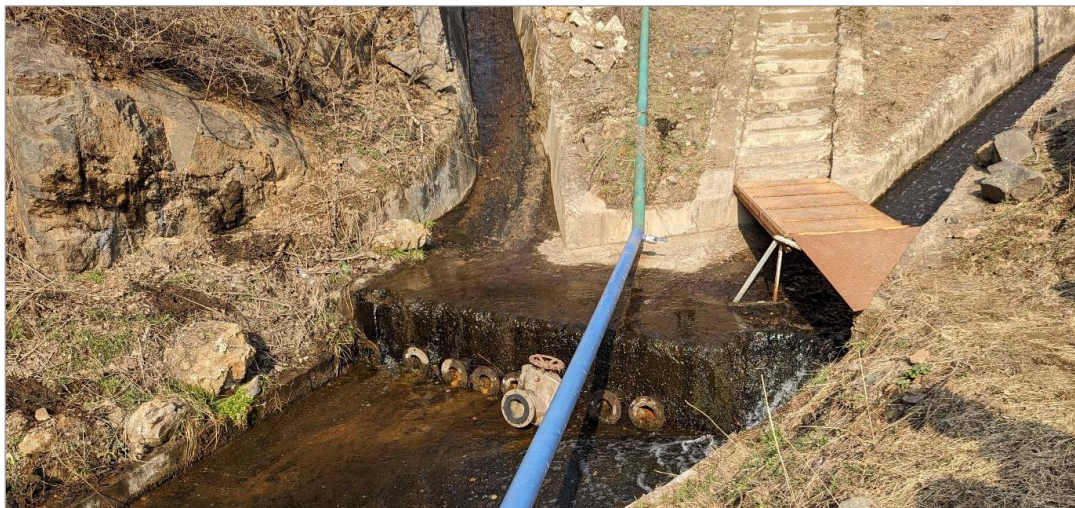
Figure 18.6 Upstream toe drain outlet pipes – TSF2
