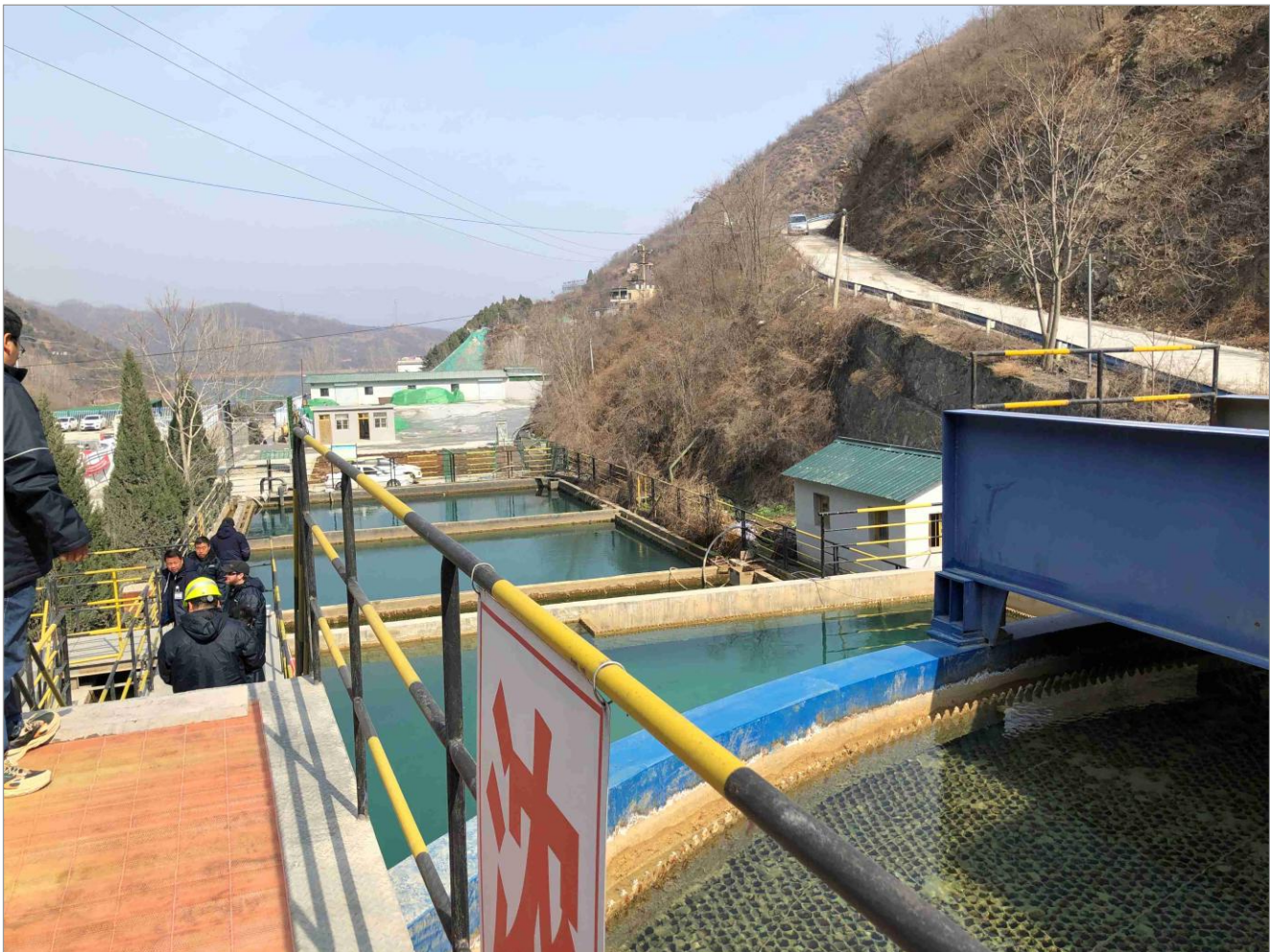
Figure 18.16 SGX water treatment plant
