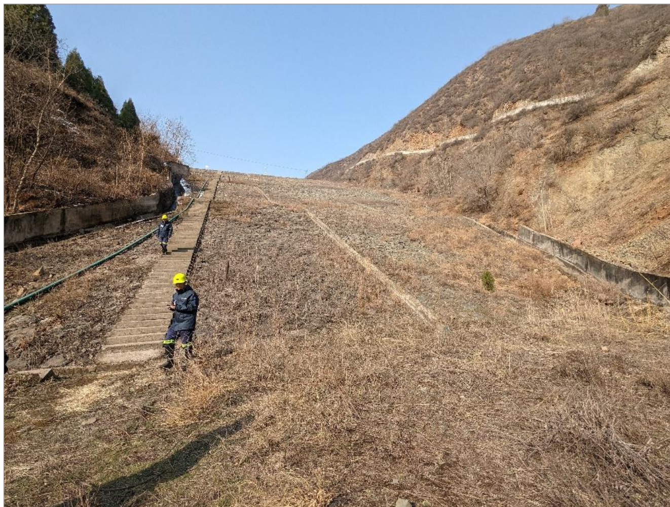
Figure 18.3 View of downstream face of TSF2 Starter Dam
