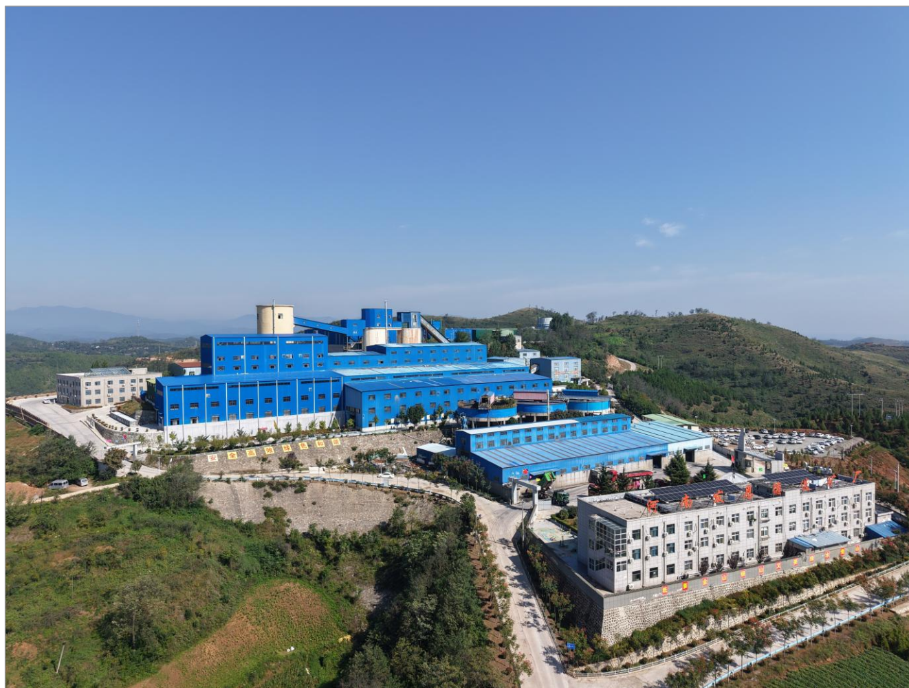
Figure 17.5 General view photos (Plant 2)
