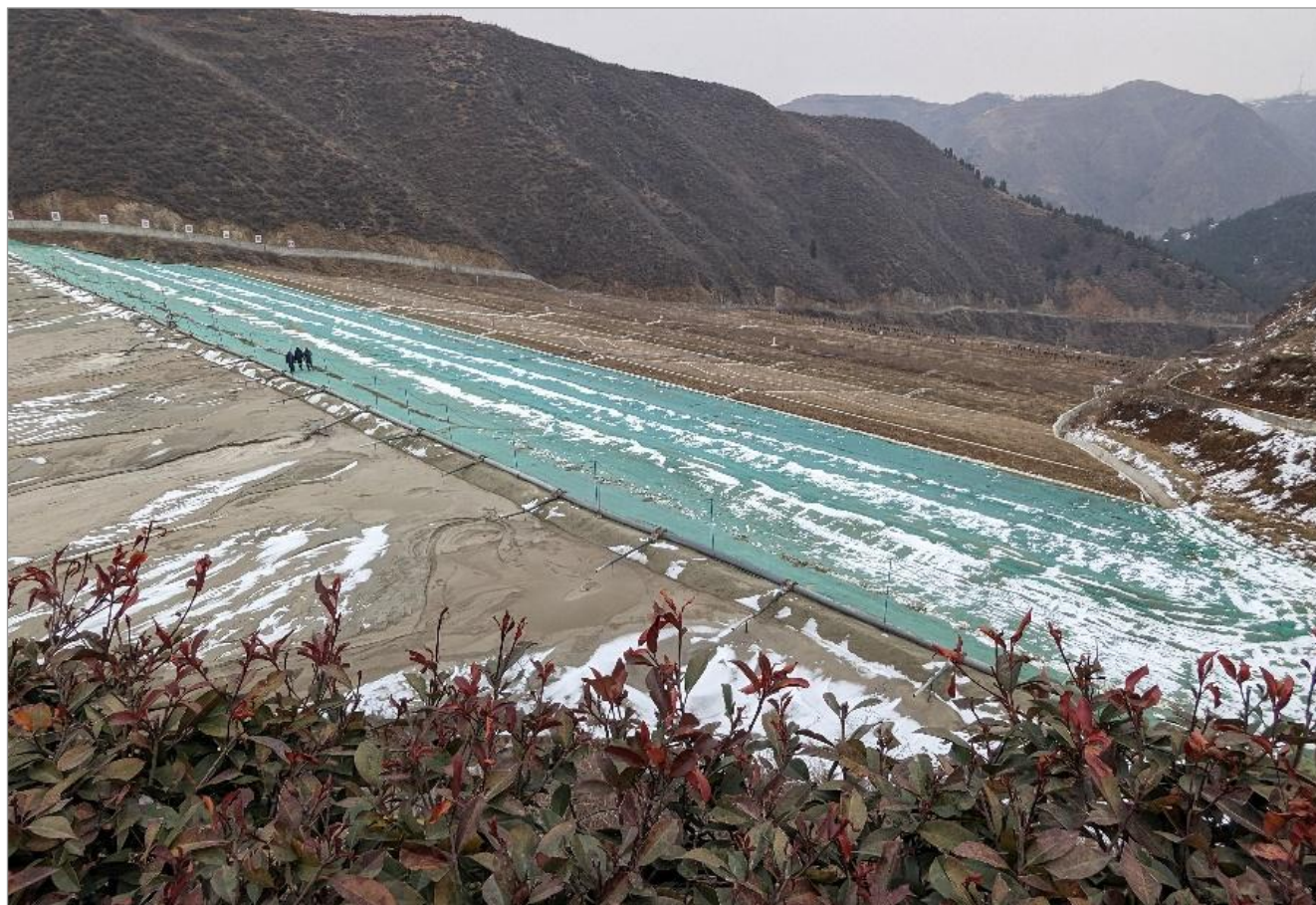
Figure 18.2 View of downstream face of TSF2
