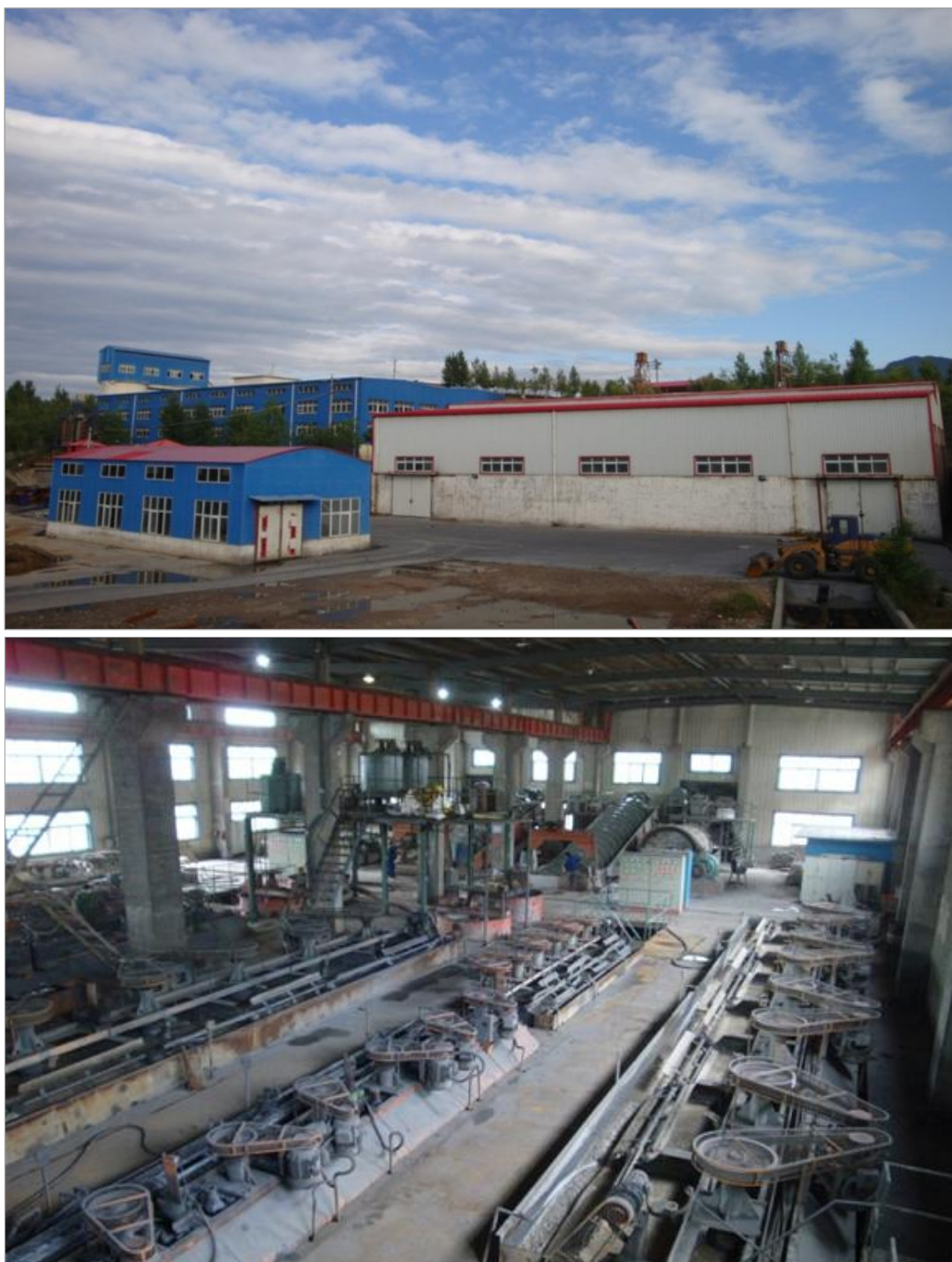
Figure 17.3 General view photos (Plant 1)
