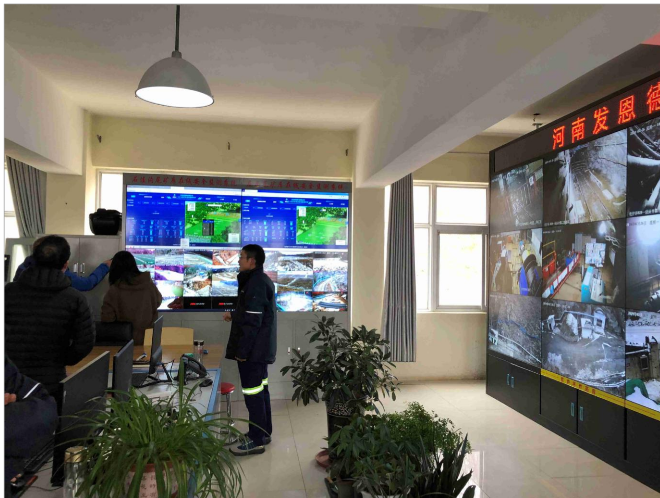
Figure 18.17 Central monitoring room
