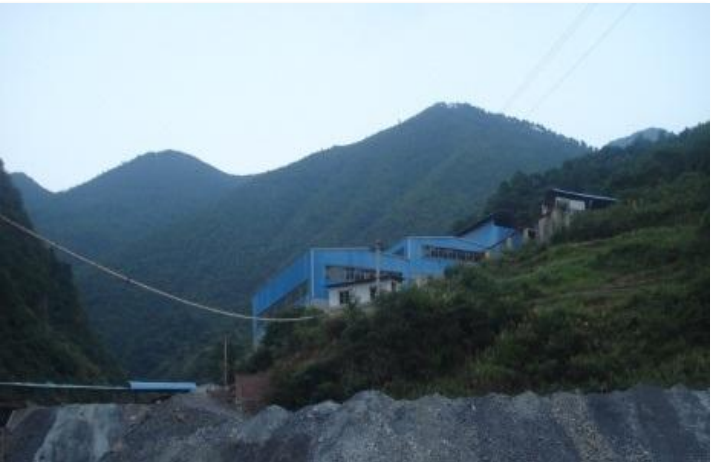
500 tpd Mill at the BYP Mine
