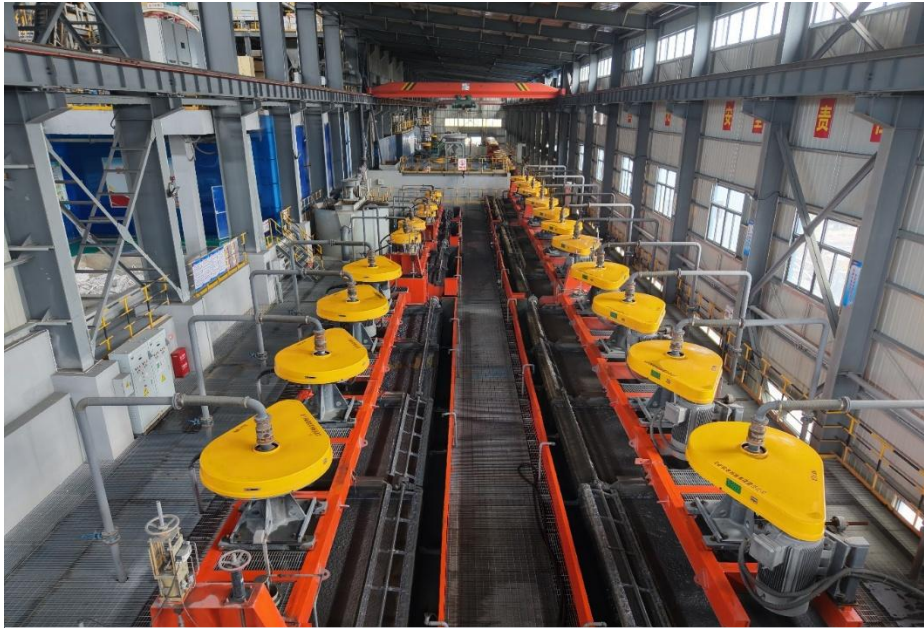
1800 TPD Flotation Line Added to Mill No. 2
