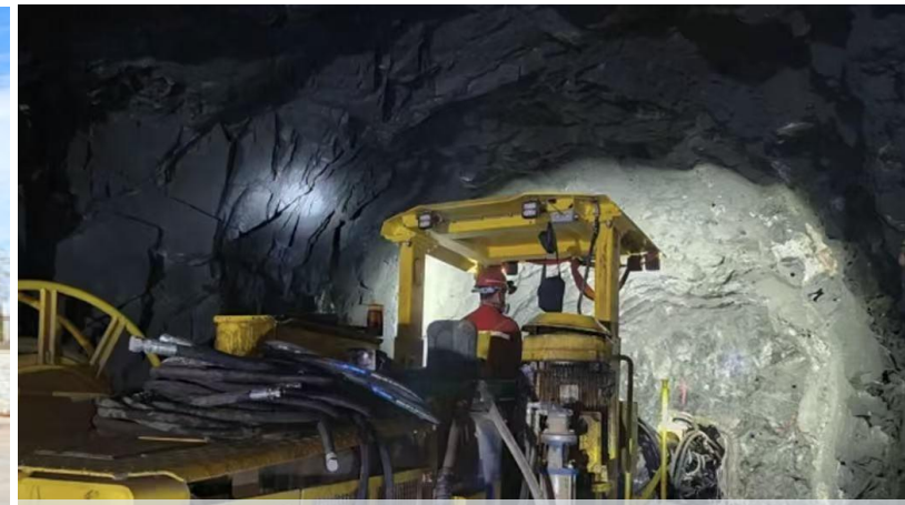
Kuanping Underground Development Underway
