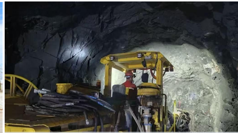
Kuanping Underground Development Underway
