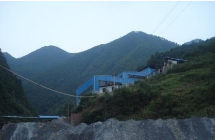
500 tpd Mill at the BYP Mine
