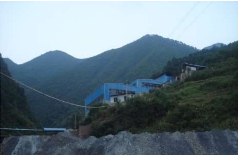
500 tpd Mill at the BYP Mine
