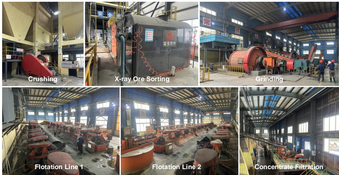
Figure 17.3: Main Production Workshop Photos of GC Processing Plant
