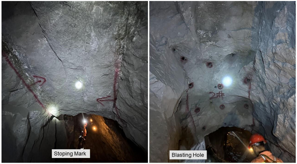
Figure 16.8: Stopping Management and Blasting Holes
