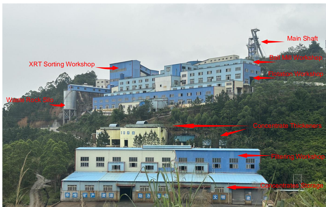
Figure 17.1: Photo of GC Processing Plant
