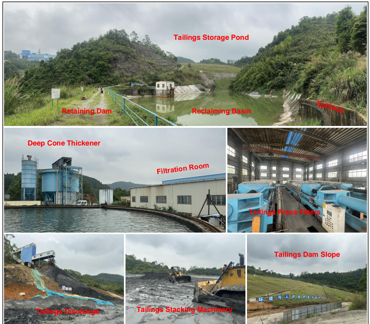
Figure 18-2: Photos of Tailings Storage Facility
