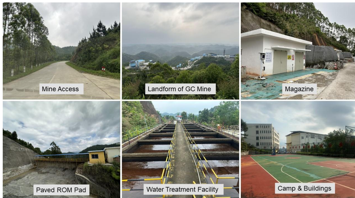
Figure 18.1: Part of Facilities of GC Mine
