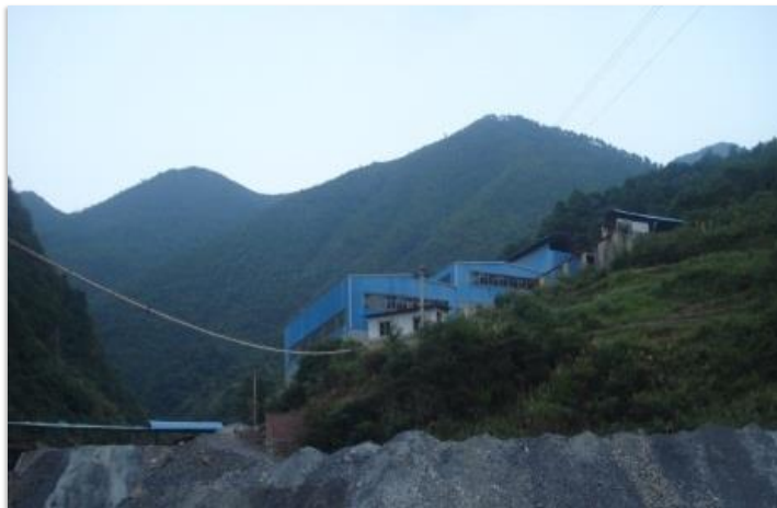
500 tpd Mill at the BYP Mine
