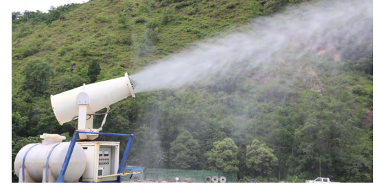
Using fog cannons to reduce dust
