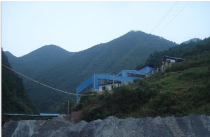
500 tpd Mill at the BYP Mine
