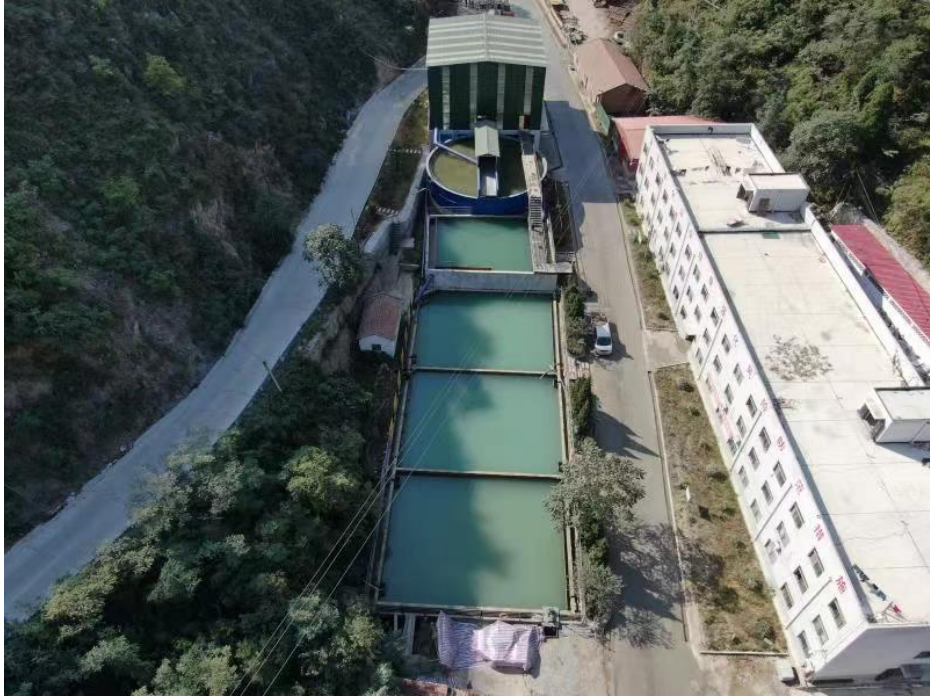
Figure 1. SGX Water Treatment Plant
