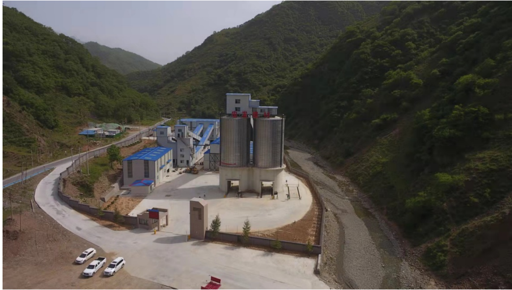
Figure 1. Ying Mining District Aggregate Plant
