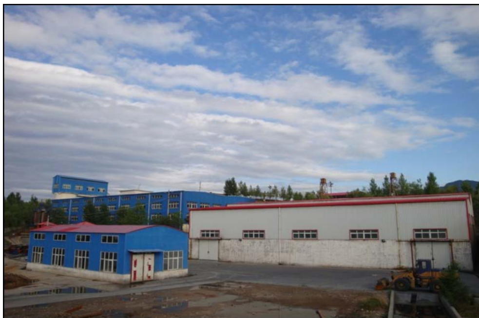
Figure 17.1 General view photos (Plant 1)
