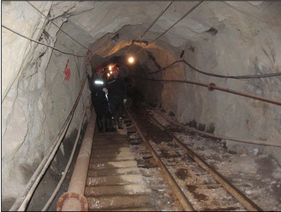
Figure 16.2 Inclined haulageway at SGX mine
