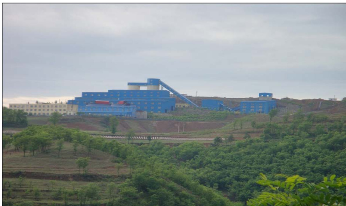
Figure 17.3 General view photos (Plant 2)
