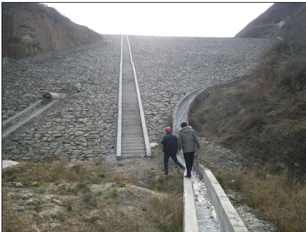
Figure 18.3 Zhuangtou TMF 1 Downstream View of Starter Dam (17 Feb 2012)
