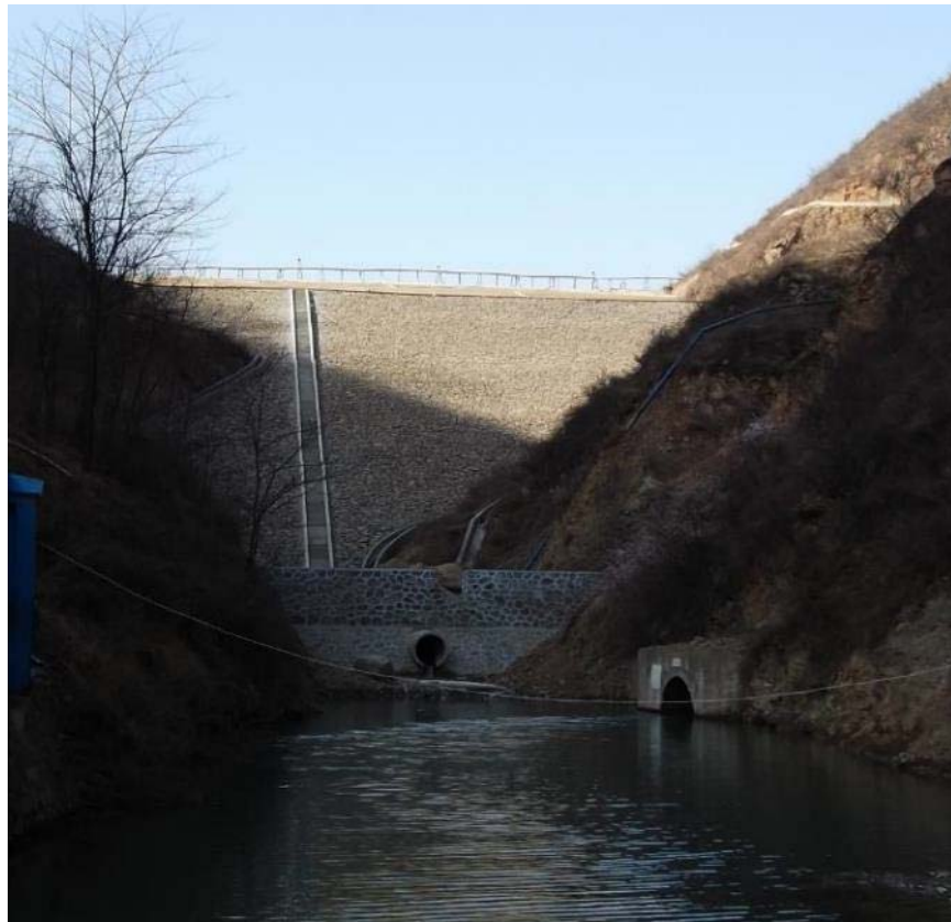
Figure 18.3 Zhuangtou TMF 1 Downstream View of Starter Dam (17 Feb 2012)
