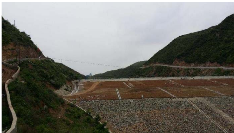
Figure 18.6 Shiwagou TMF 2 Downstream view of starter dam (14 May 2014)
