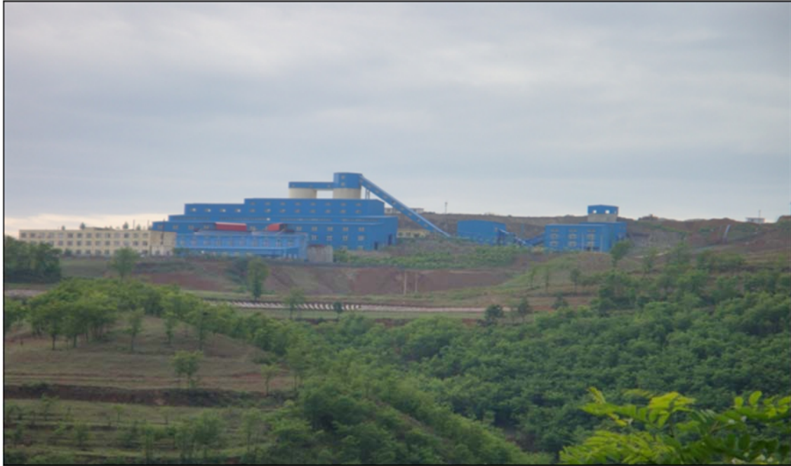
Figure 17.5 General view photos (Plant 2)
