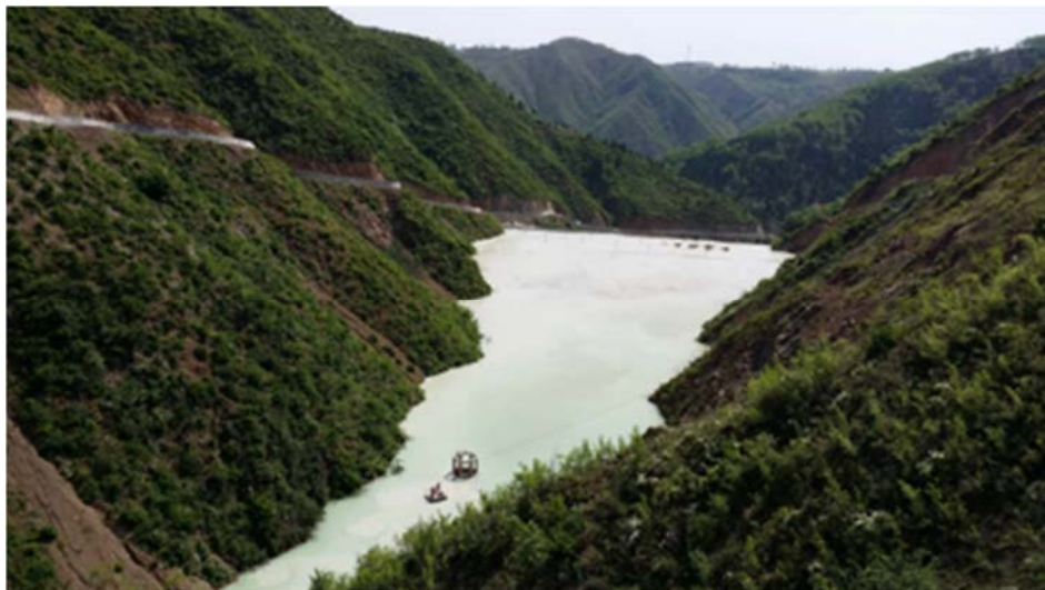
Figure 18.5 Shiwagou TMF 2 Upstream view (12 May 2014)
