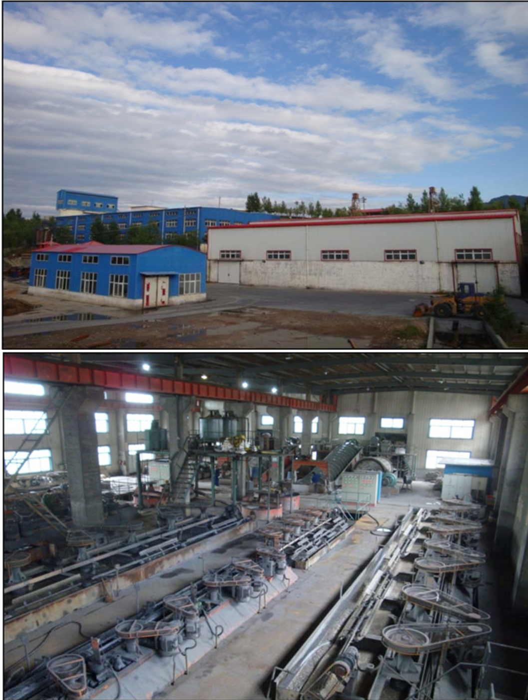
Figure 17.3 General view photos (Plant 1)
