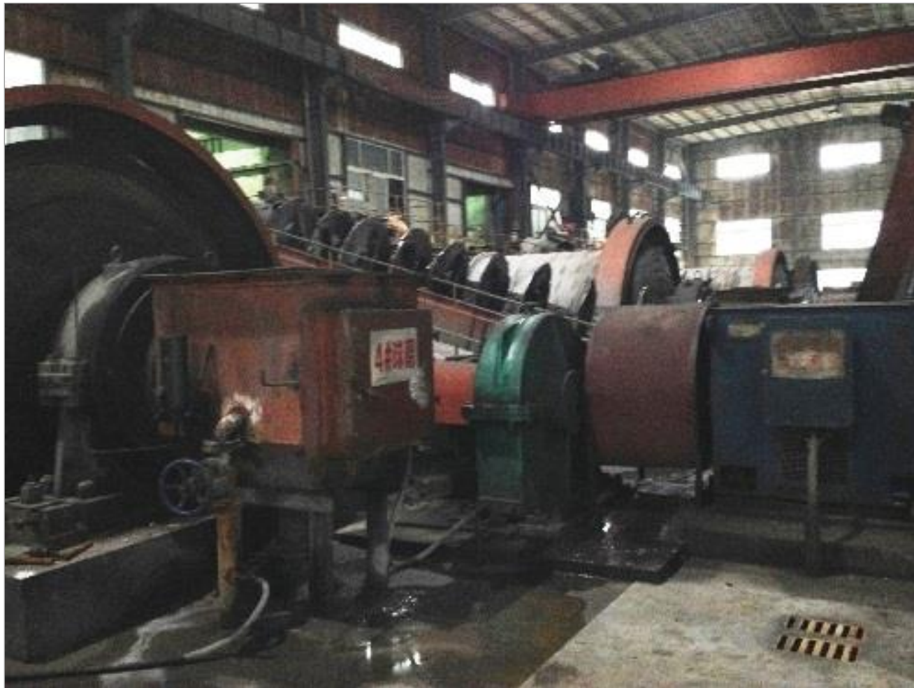
Figure 17.4 Grinding mills and spiral classifier
