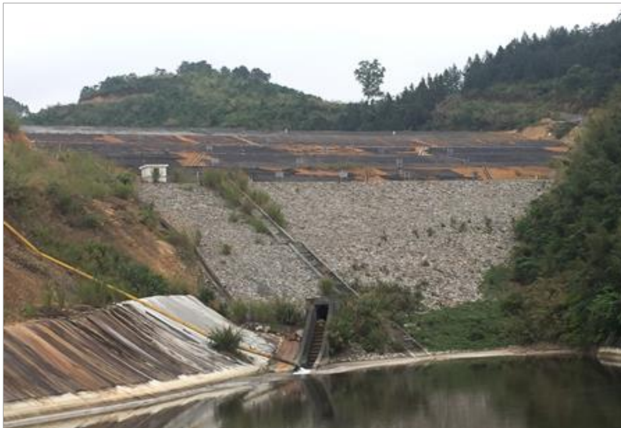
Figure 18.3 GC TMF dam and water seepage
