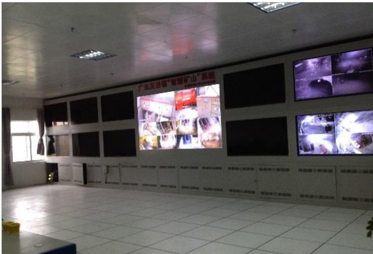
Figure 17.8 Control room screens
