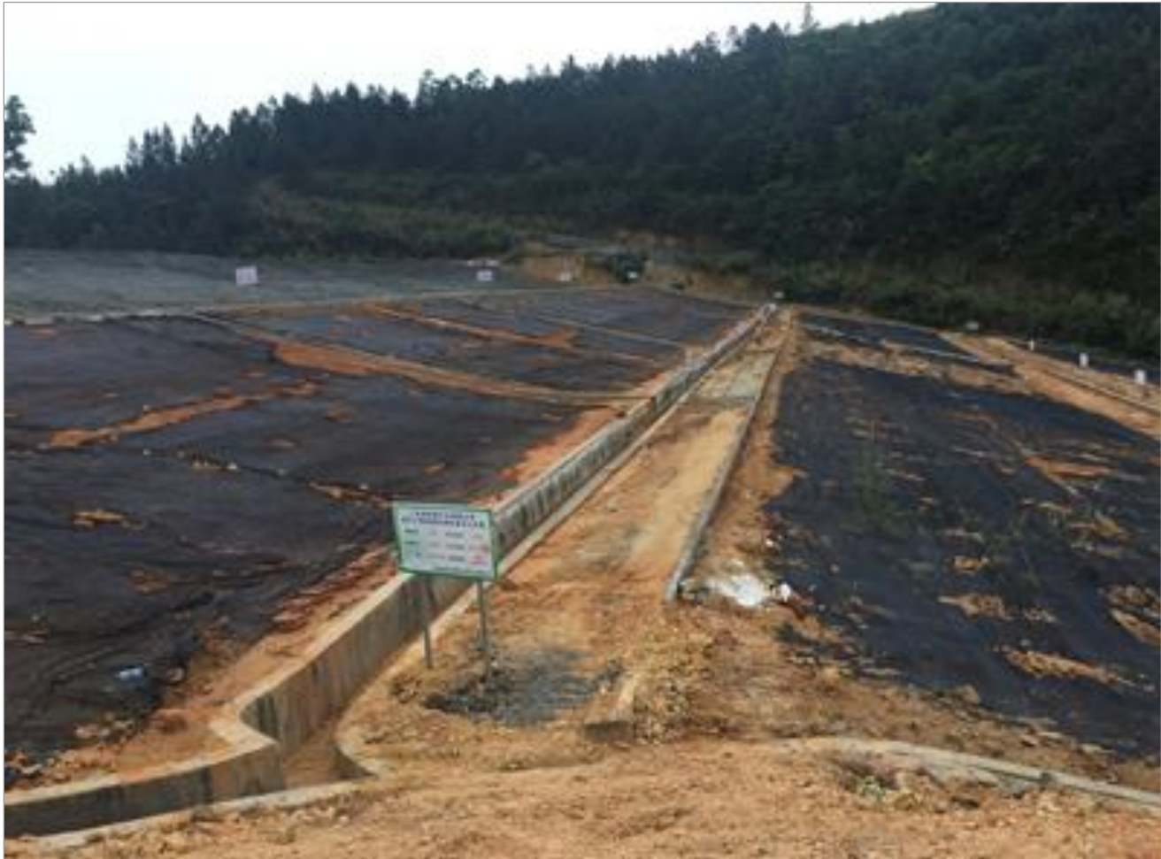
Figure 18.4 TMF dam water catchment
