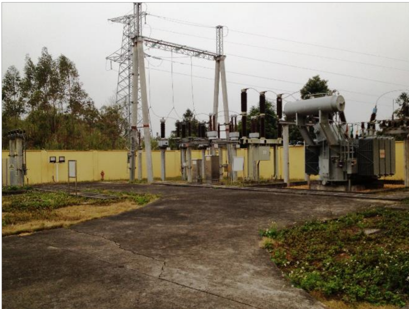
Figure 18.6 GC mine substation
