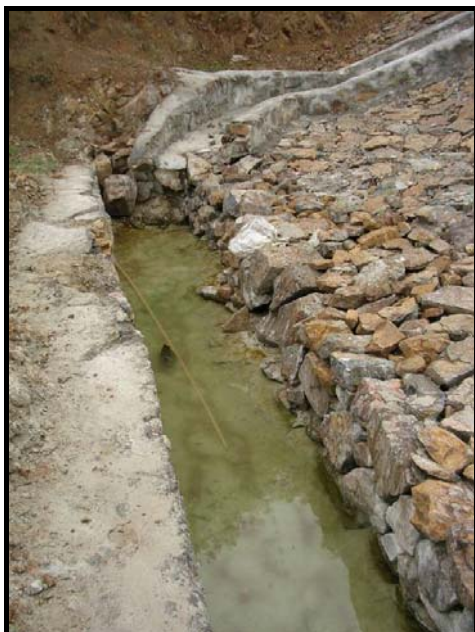
Figure 6-4: Moderate Seepage at Downstream Toe of Starter Dam
