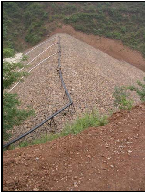
Figure 6-3: Zhuangtou TSF Starter Dam (14 June 2007)
