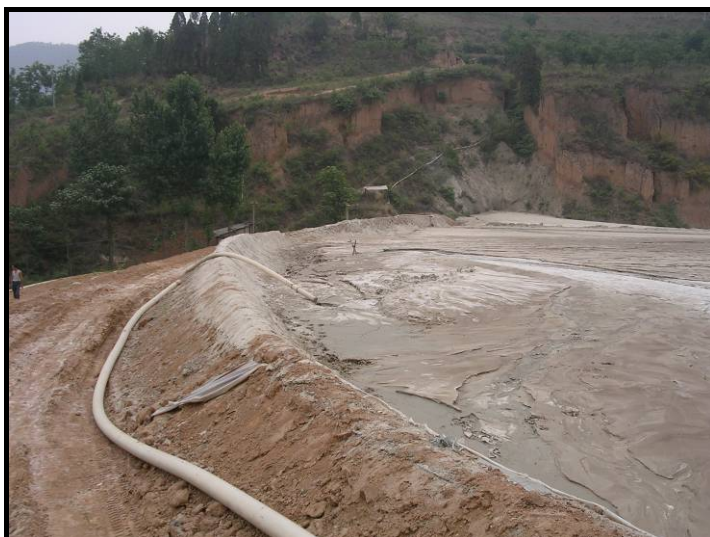
Figure 6-6: Discharge of Tailings into Dong Zi Gou TSF (16 June 2007)
