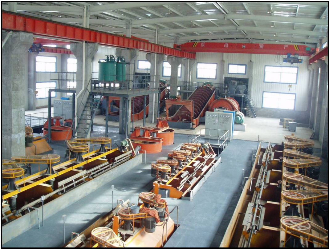
Appendix 16-2: Milling and flotation Setup of No.2 Mill
