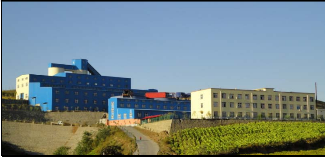
Appendix 16-1: General View of No.2 Mill
