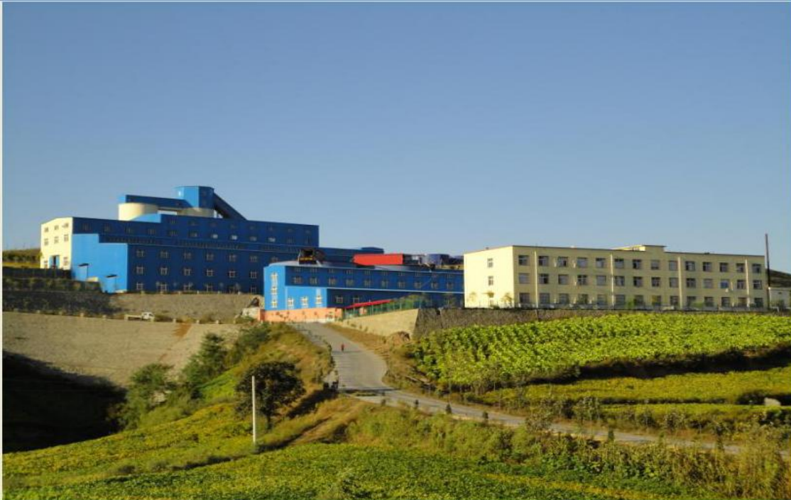
Appendix 16-1: General View of No.2 Mill
