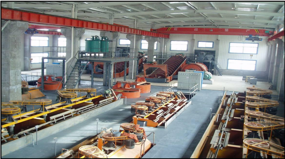
Appendix 16-2: Milling and flotation Setup of No.2 Mill
