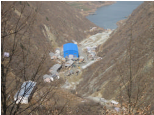
Photo 2: View from the hill-top of the camp and steel-framed warehouse
