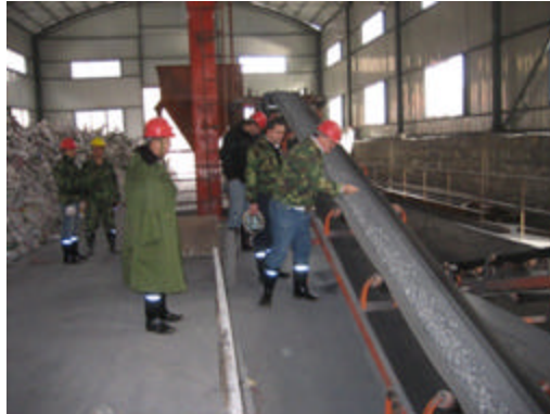
Photo 3: Crushing circuit for direct shipping ore
