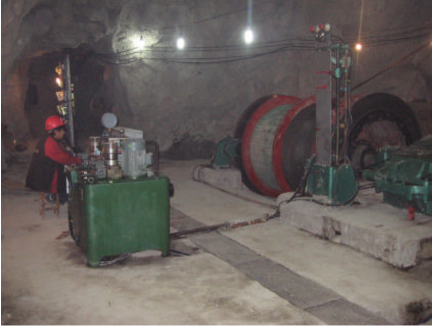
Photo 1: Hoist chamber of No. 3 shaft in adit CM101
