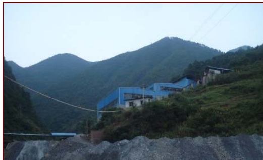
500 tpd Mill at the BYP Mine
